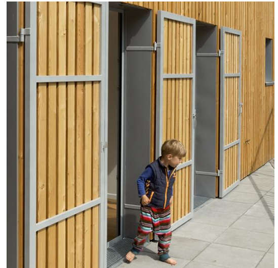
Larch slatted wood shutter Steel frame
