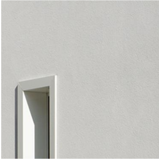
White plaster (north façade body)
