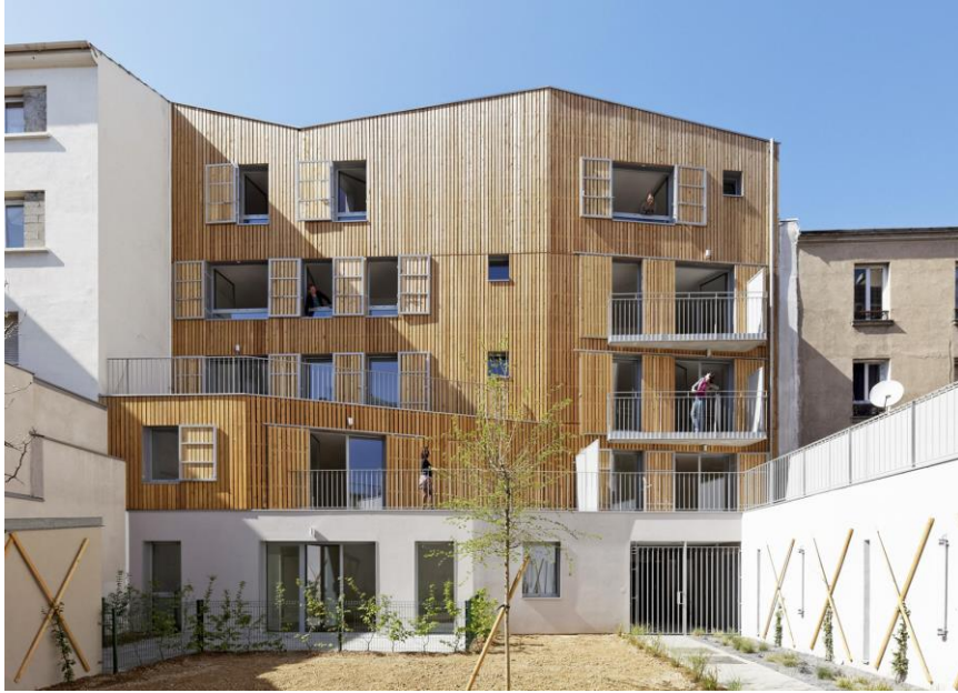
New build wooden façade
