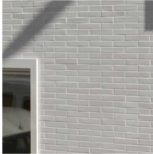
White varnished brick (north façade base)
