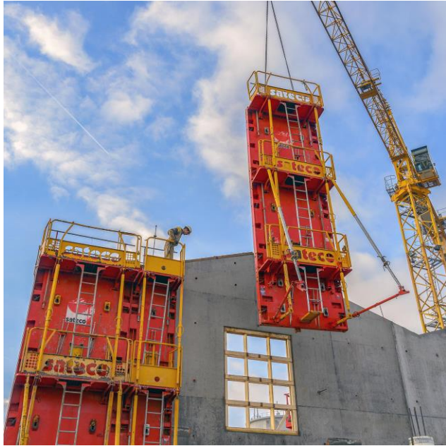
Form concrete walls
