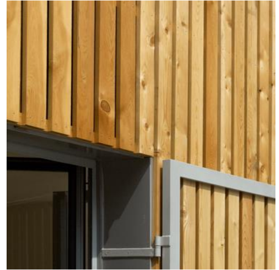
Larch slatted wood covering (south façade)
