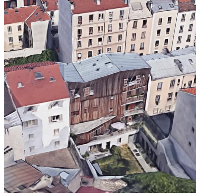
Rain, wind and sun effect on the non protected façade
