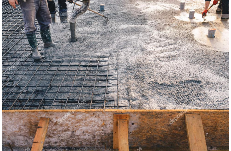
Poured concrete slab
